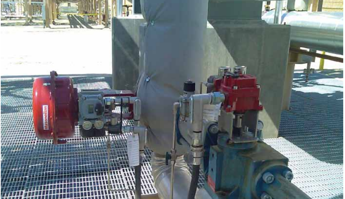
SVI II AP positioner on single acting control valve
